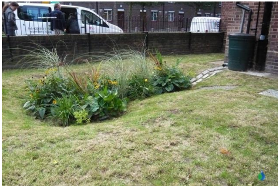
Fig 26 Raingarden within housing garden
